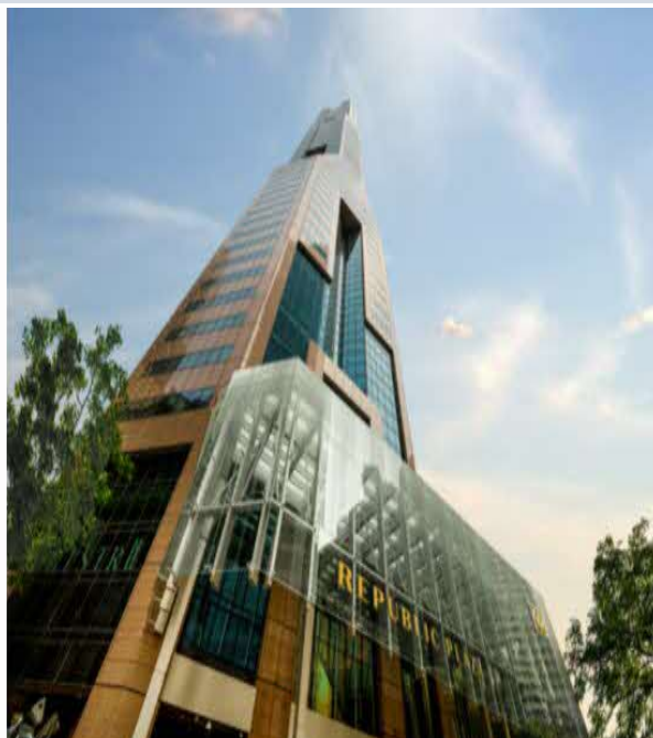
Republic Plaza - 280-m tall flagship building, CDL's HQ
