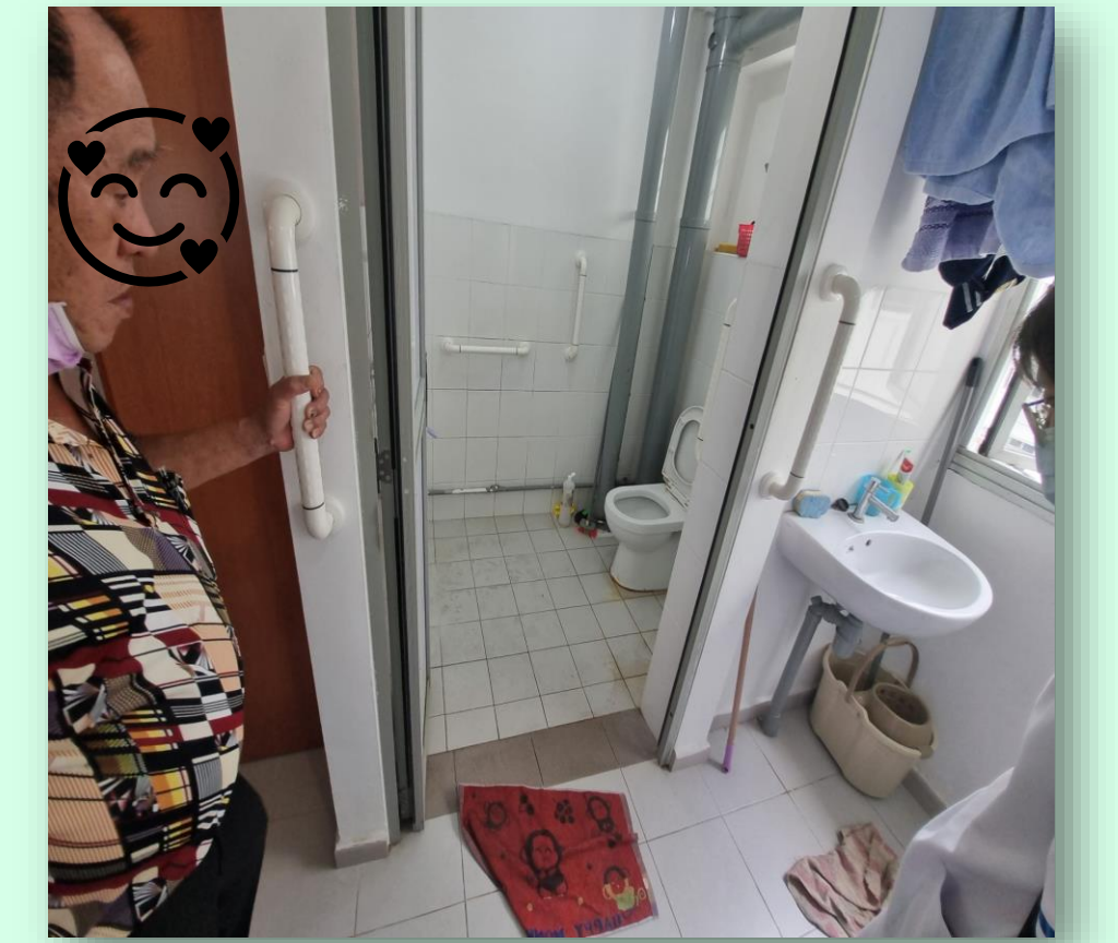
Toilet grab bars inside toilet and its entrance (these were fixed prior to last hospital admission); placement of non-slip mat outside toilet
