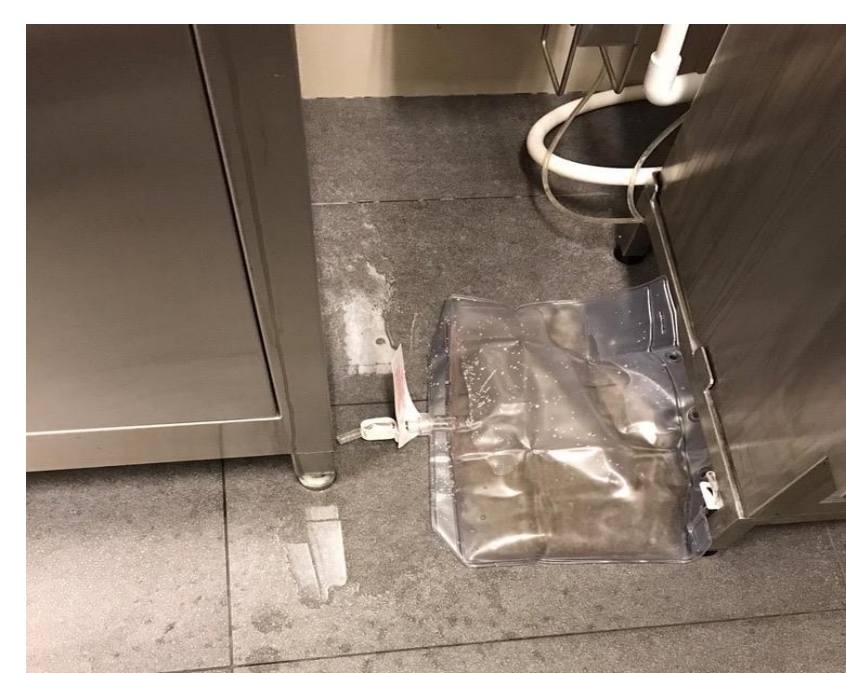
Picture 2: Spillage of effluent bag on floor
