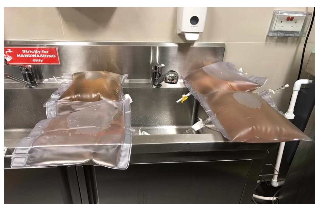
Picture 1: Effluent bag placed at side of sink.
