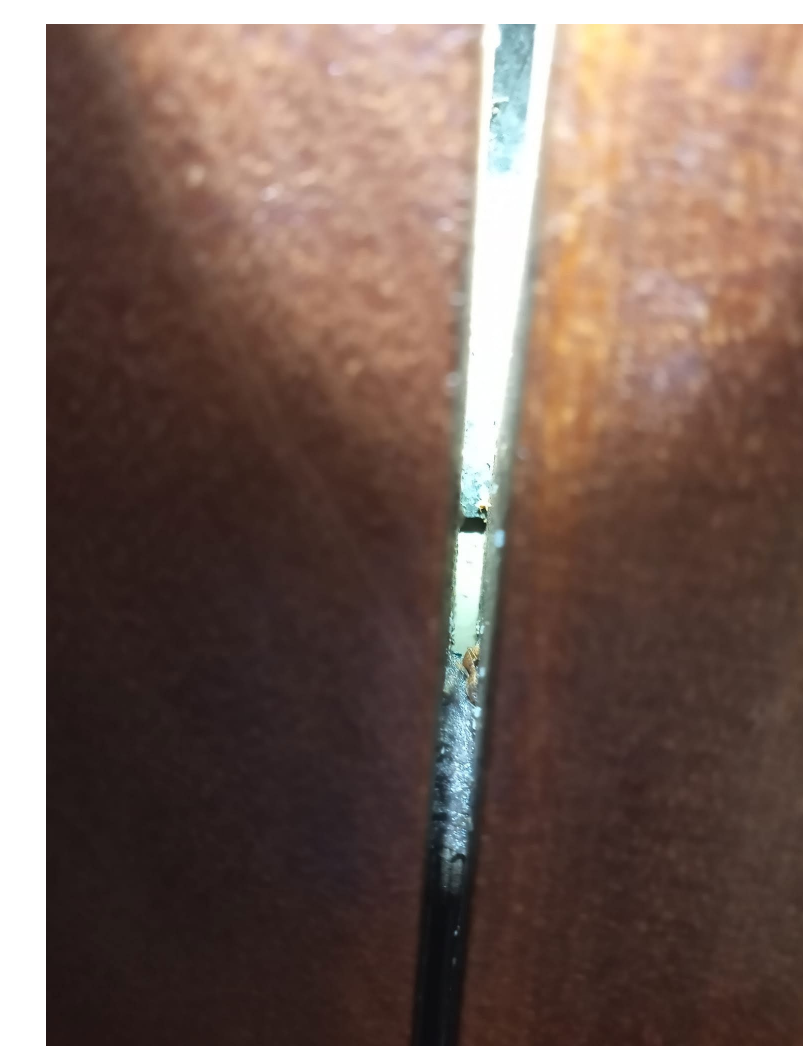
Pest harborage in gaps and crevices
