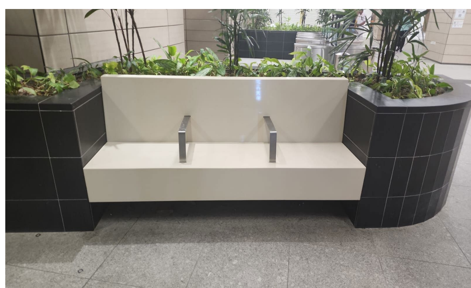
Benches restored with seamless design using polished quartz
